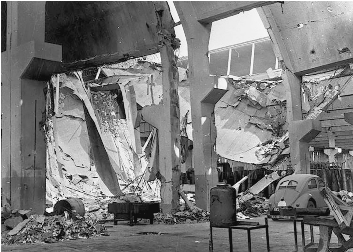
Allied raids on the Volkswagen factory caused roofs to cave in and walls to collapse, as in this photo from 1944, but most of the machinery survived, and production was only temporarily interrupted. ( Volkswagen Aktiengesellschaft )
