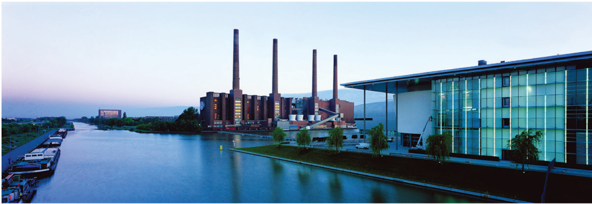
A view of the main factory in Wolfsburg on the banks of the Mittelland Canal in 2007. In the foreground is the entrance to the Autostadt, a museum and temple of auto worship. ( Collection ullstein bild, Getty Images )
